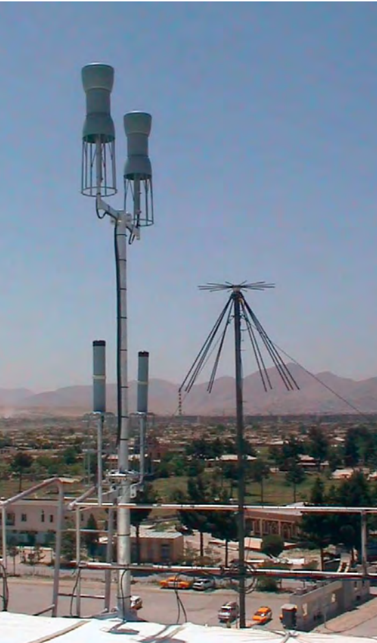
FIG 2 The R&S®HK012 and R&S®HK014 antenna systems at Kabul airport.
