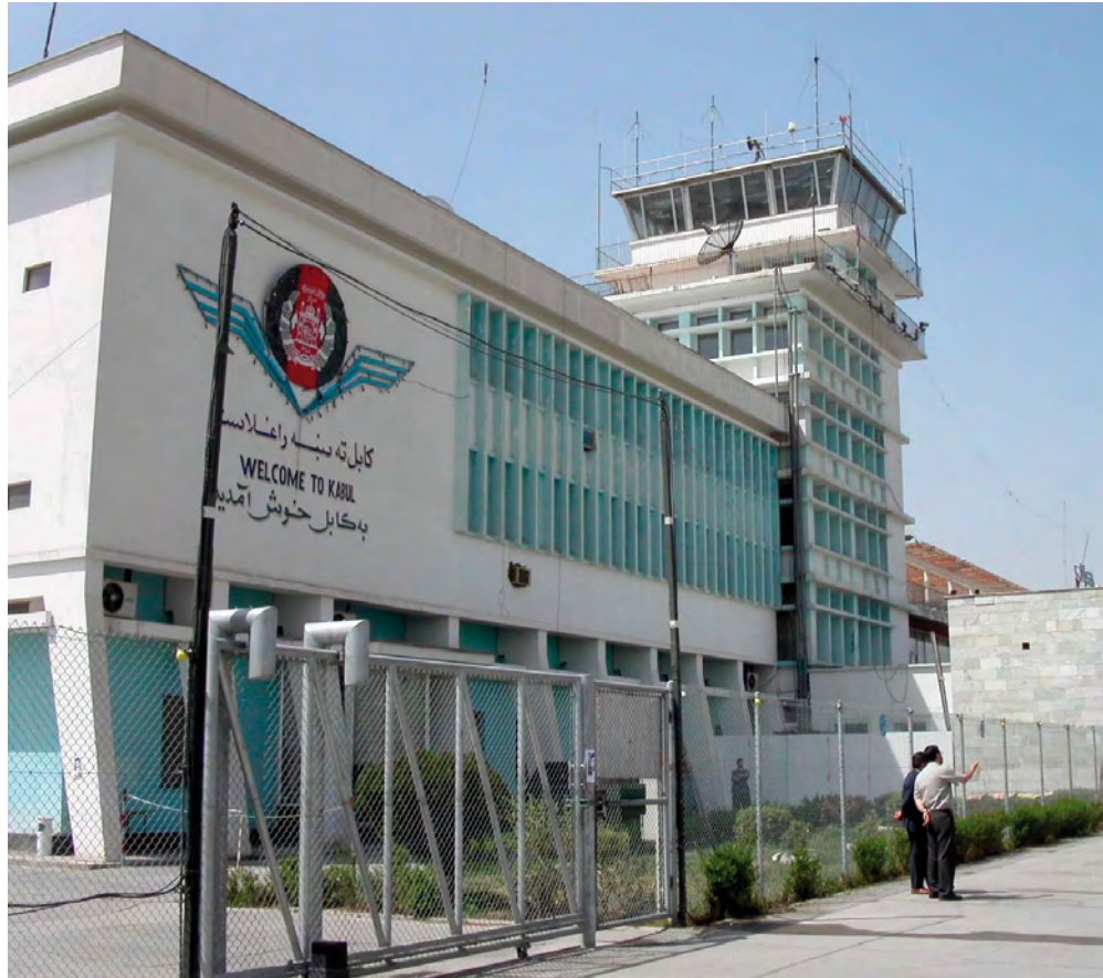
FIG 1 Tower building at Kabul airport: Communications technology from Rohde&Schwarz ensures air safety.
